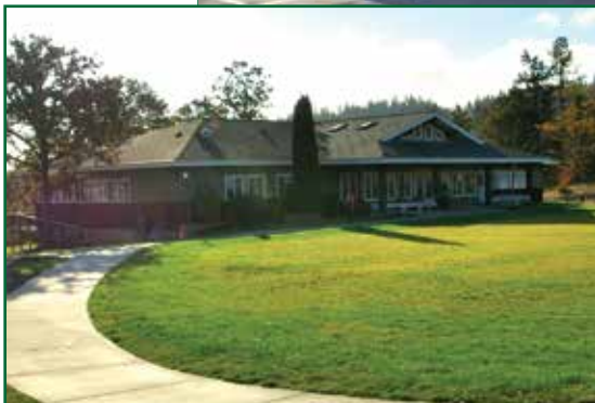
The McDonald Building (left) sees high usage as it is the location of the OHS 6th grade, MS Math, MS Social Studies, and MS Language Arts in addition to all Upper School Foreign Languages (Mandarin, French, and Spanish).
